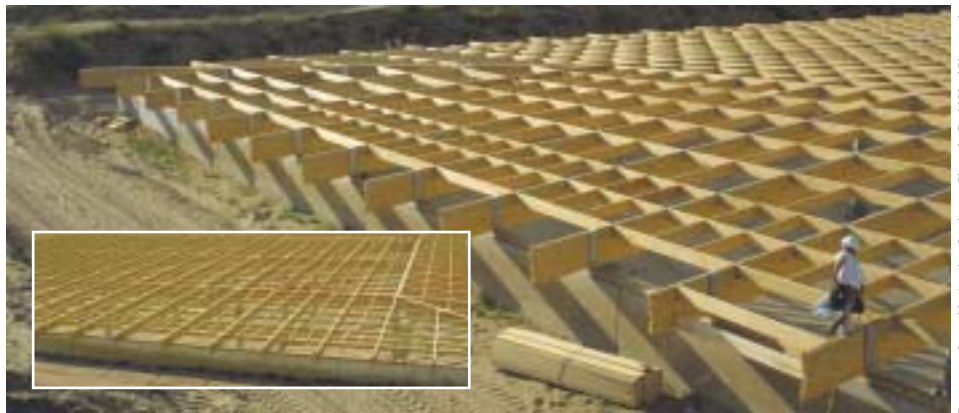
Glulam Yellow cedar beams and trusses frame roof over 5.3 hectare water reservoir.
